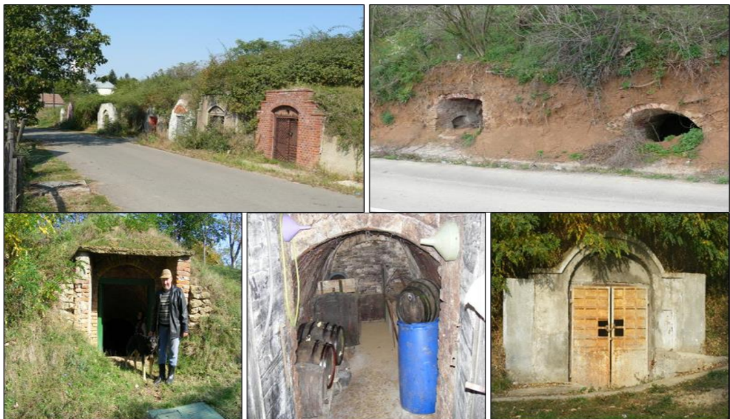
Figure 10. Independent cellars of households in the villages of Paleu (top left), Sîșterea (middle), Tăutelec (top right and bottom left), and Cetariu (bottom right)
